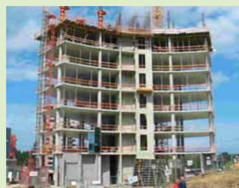
Office building, Tallinn, Estonia
