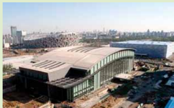
Olympic hall, Beijing, China
